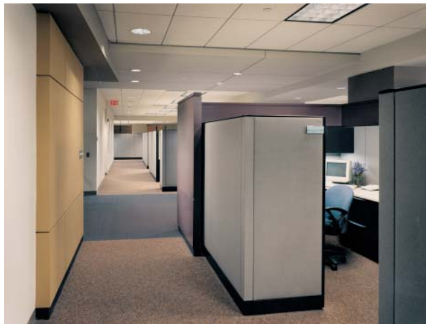
This accent wall with simple gypsum board reveals, creates a pattern, which provides the illusion of wall panels. The change in carpet tile and a drop in the gypsum soffit at the corridor serve as a wayfinding tool. The soffit also has reveals that visually break up the solid gypsum plane.
