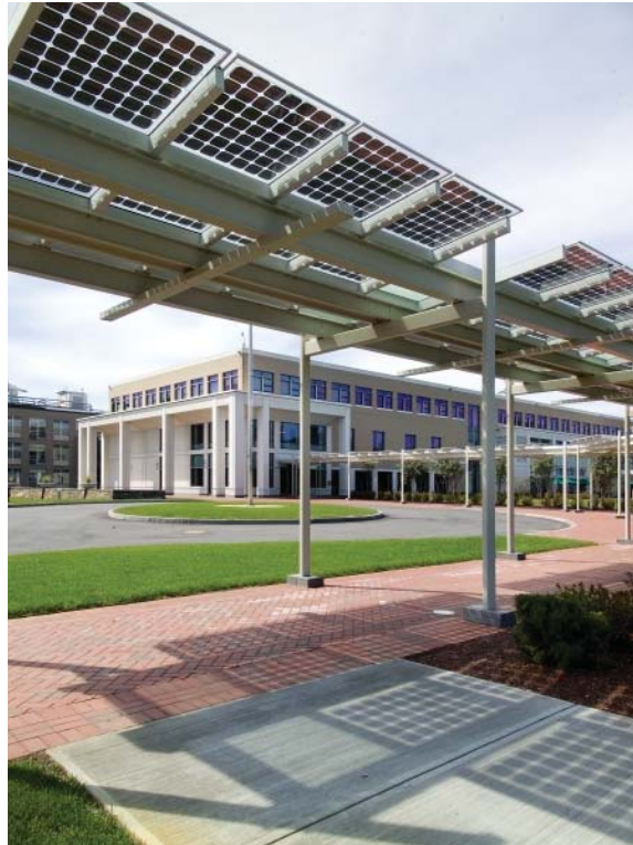
Sustainable design features reduce operating costs and help the LEED Silver MITRE Center attract and retain talented employees. Photo by Peter Vanderwarker.
