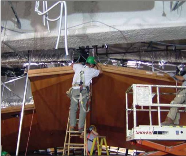
Construction photos showing installation of wood panels. BIM helped avoid duct/steel/millwork conflicts.
