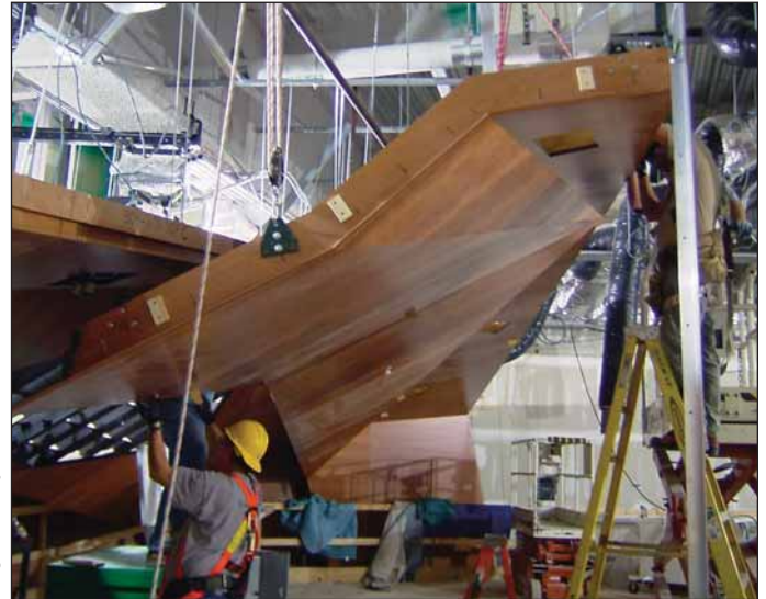
Construction photos showing installation of wood panels. BIM helped avoid duct/steel/millwork conflicts.
