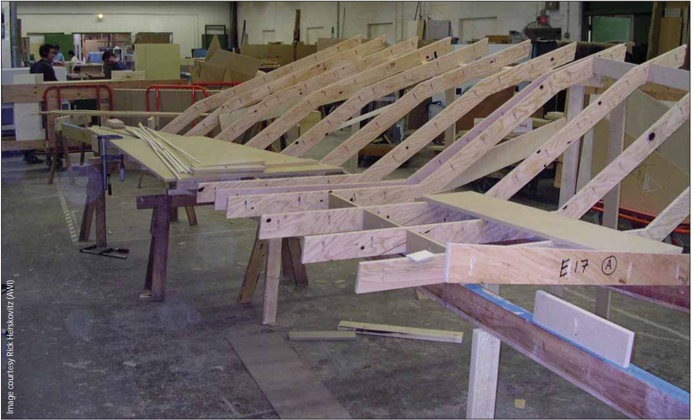
Full-scale mockup made from BIM model. The design/construction technique can help minimize tolerance-related problems.
