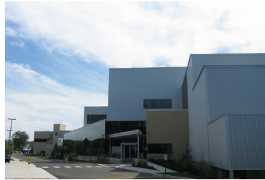
Photos courtesy of KlingStubbins
