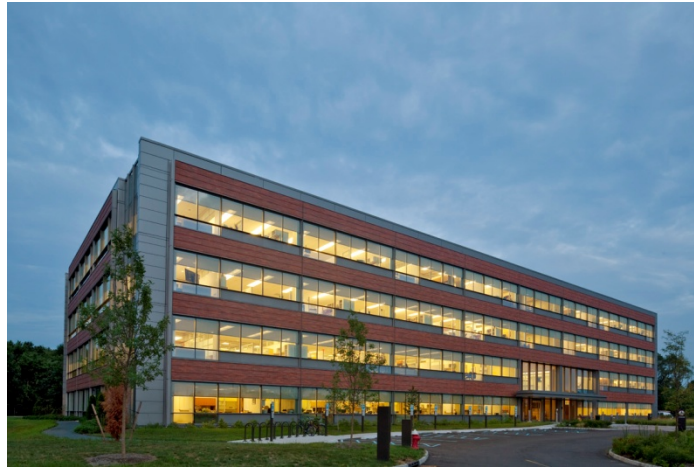
Designed by KlingStubbins, Boston Properties' Carnegie Center West in Princeton, New Jersey, earns LEED Gold Certification. Photograph courtesy of Eduard Hueber/archphoto.com
